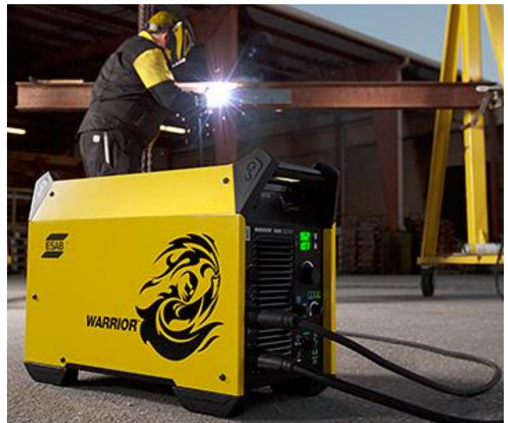
MMA welding using Warrior 400i CC/CV
